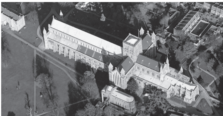
Figure 8. A pictometric slanting image shows facades of the buildings and their height (Source: Geo Info Strategies)
